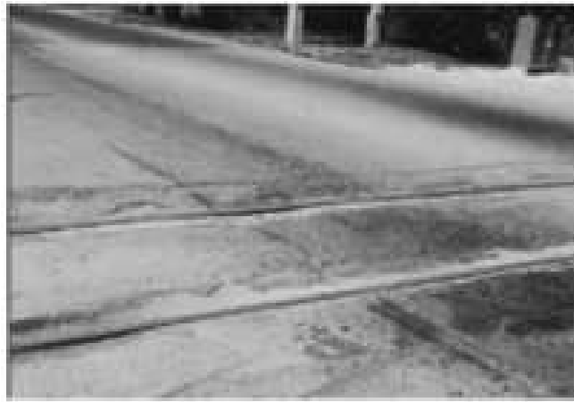
Gambar 2.32 Rusak Perpotongan Rel ( Railroad Crossing )
