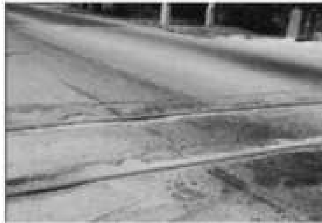
Gambar 2.32 Rusak Perpotongan Rel ( Railroad Crossing )
