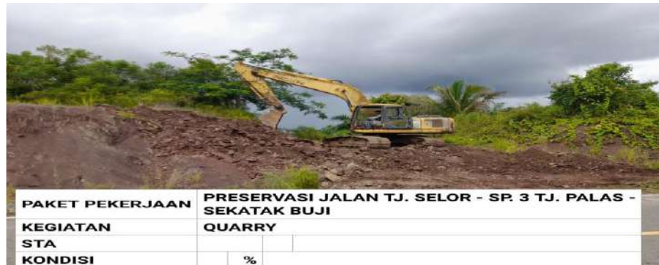
Gambar 2.1 Excavator (PT. Cahaya Baru Prima )
