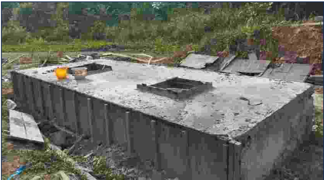
Dokumentasi pekerjaan ground water tank
